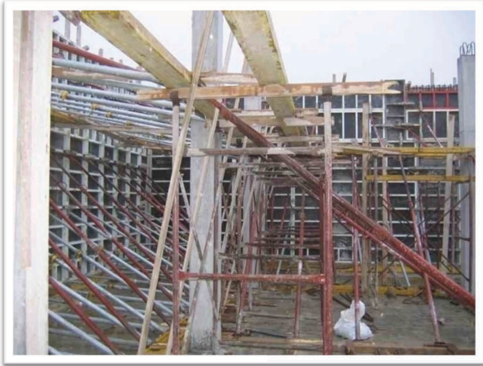
Picture 20: Support for Formworks in Reservoir. (Photo: ADA Project Archive)
