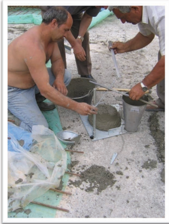
Picture 30: Workers performing concrete slump test. (Photo: ADA Project Archive)
