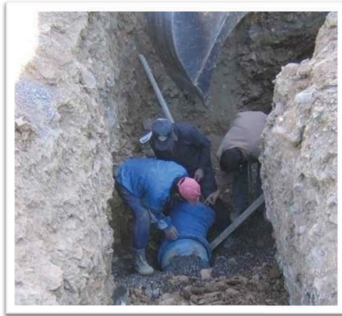
Picture 17: Workers installing a pipe connection. (Photo: ADA project archive)
