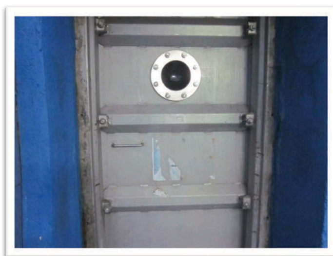
Picture 3: Bull-Eye window in steel pressure door. (Photo: C. Stubenberg)
