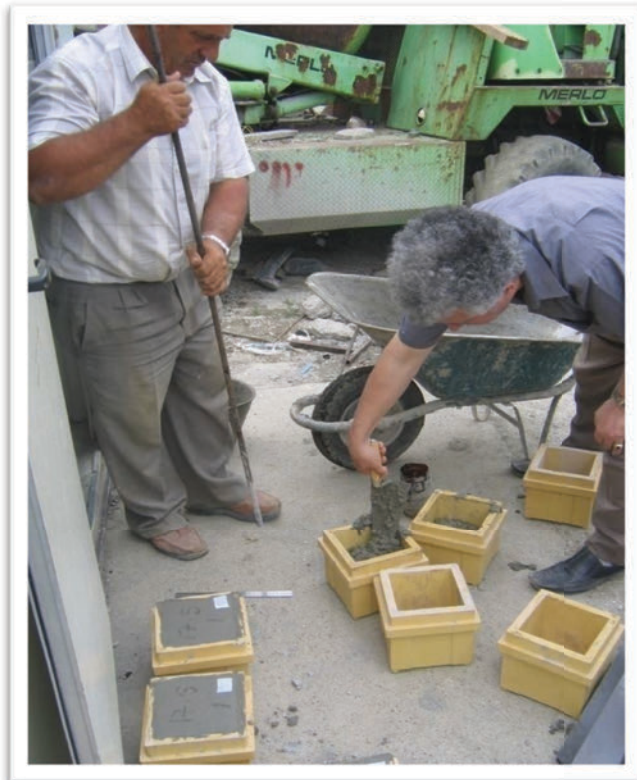
Picture 32: 15x15x15cm Testing cubes are casted (Photo: ADA Project Archive)
