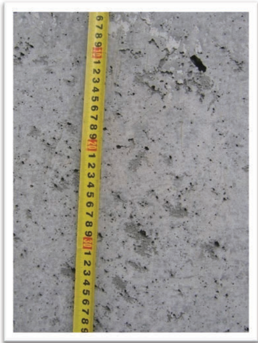
Picture 26: Pores in the Weisse Wanne measured with ruler. (Photo: ADA Project Archive)
