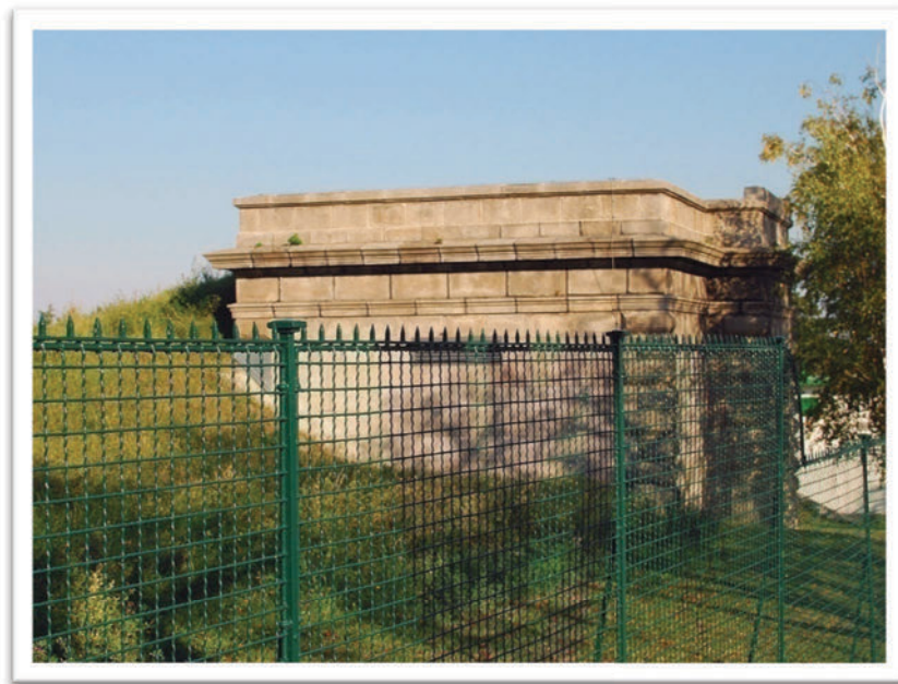
Picture 19: Control room of a Viennese water reservoir on the Schafberg. (Photo: Winterleitner Heinz)
