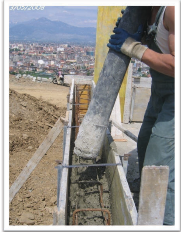
Picture 31: Pouring concrete into the formworks. (Photo: ADA Project Archive)
